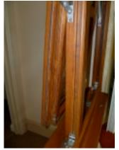
The wood effect textured finish for example has a major advantage over woodgrain pvc in that it is not a foil and unlike pvc, coats every surface of the window profile.
